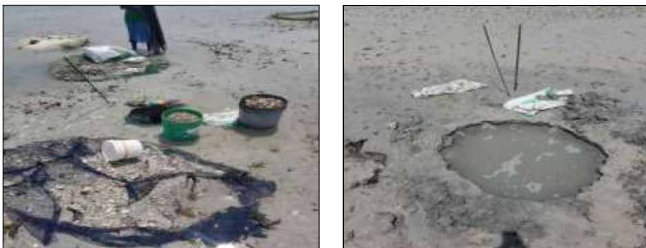
Figure 5: Dredging activities along Mikadi Beach
